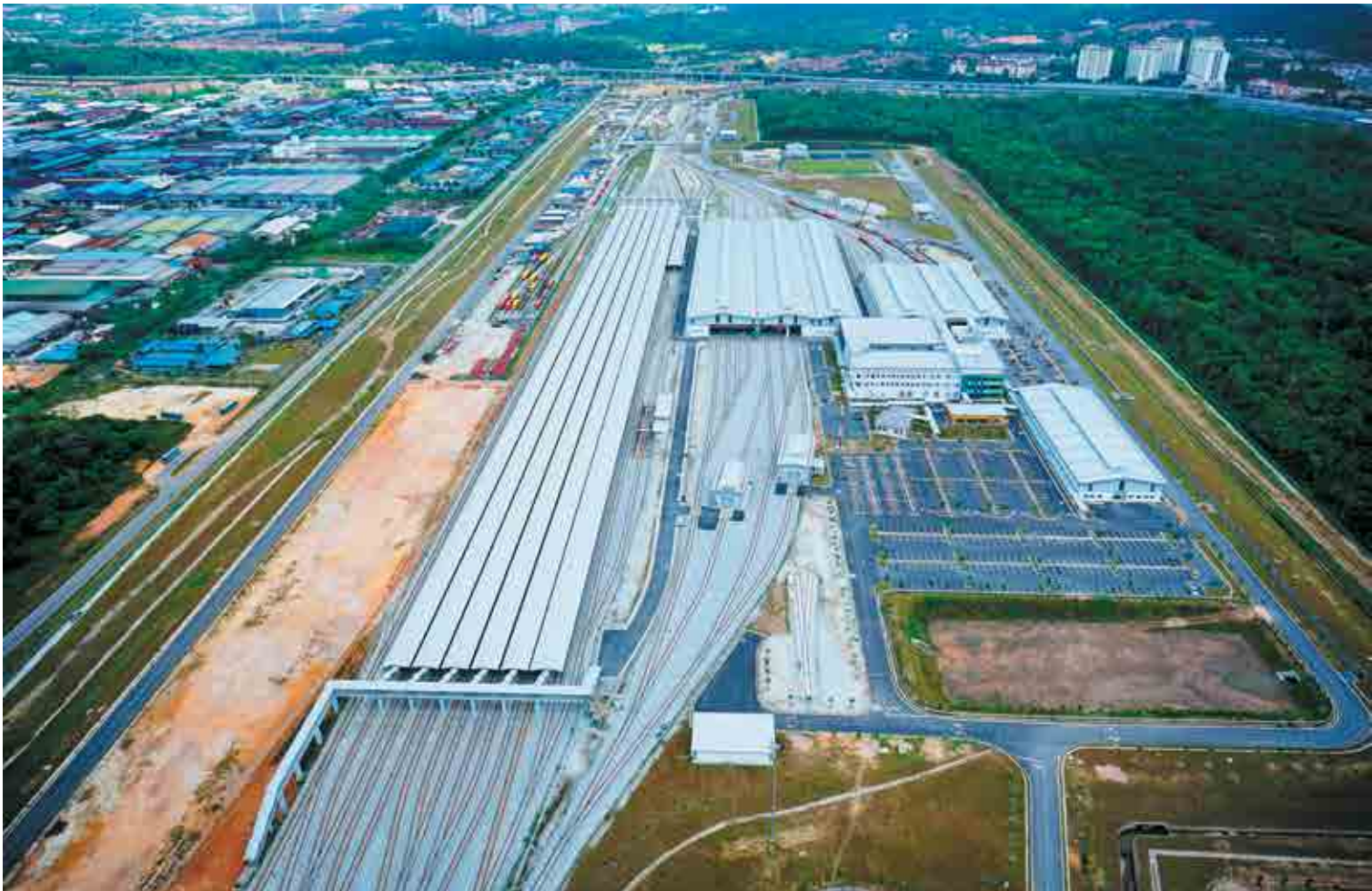
At 162 acres, the KVMRT Line 1 - Sungai Buloh Depot is the biggest train depot in Southeast Asia. It is able to house 100 trains.
