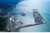
Seawall-Taipei Port is Gamuda's second project in Taiwan. It involves the construction of a 4,014-metre-long seawall for a reclamation project in the logistics storage area of Taipei port, dismantling existing 945m of seawall structures, and Southport shore protection works.
