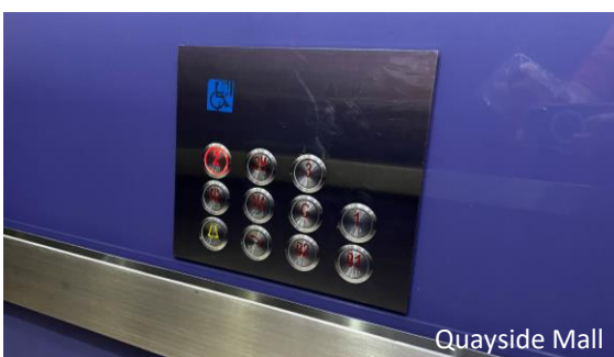
Elevator button with the braille feature and positioned at waist-level
