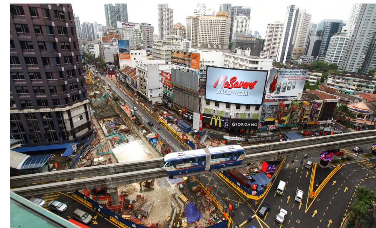
Constructing in an bustling city centre, we ensured business and utility services continuity in the area.
