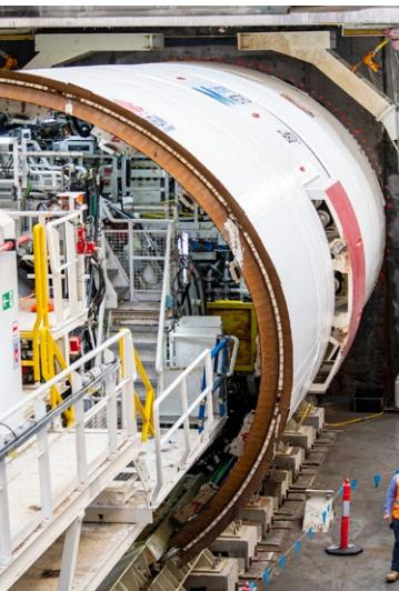
Gamuda launched TBM Betty and TBM Dorothy, Australia's first autonomous tunnel boring machines (TBMs). For the first time in Sydney Metro history, TBMs Betty and Dorothy will use non-potable water to excavate and cool themselves.
