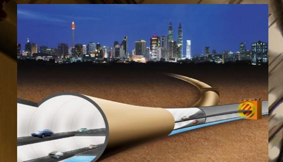
**The world's first dual-purpose stormwater diversion and motorway tunnel**
