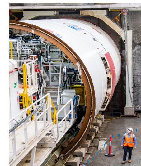
Largest overseas tunnelling contract
