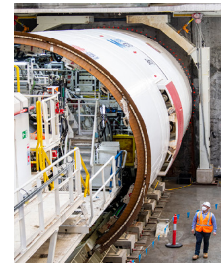
Largest overseas tunnelling contract
