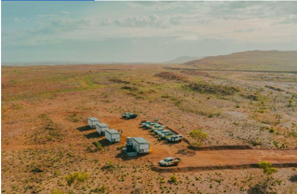
Caption: Early site works for the Jinbi Solar Farm.
