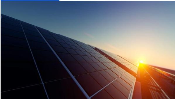
Caption: A stock image representing the Jinbi Solar Farm. The landmark development will feature 160,000 solar panels, marking a significant step forward for renewable energy in Western Australia and the decarbonisation of the Pilbara region.
